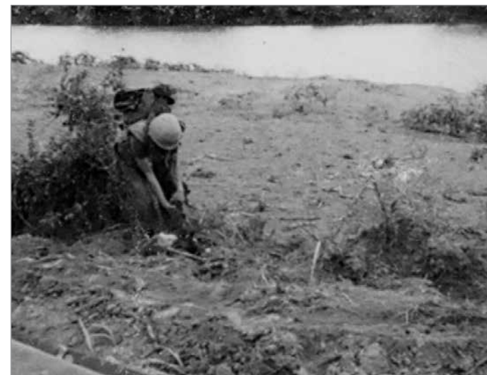
Dig 'em out of the trench line
